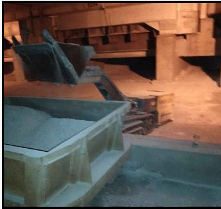
Figure 1. Mini dozer cleaning the basement.
