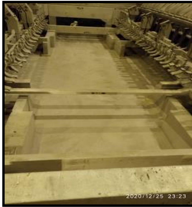
Figure 2. Clean pot site in the basement.
